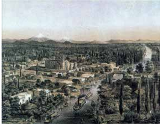
Picture of the canal “before”
